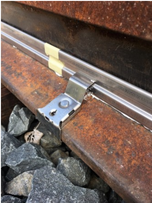
The nVent rail switch heating system
