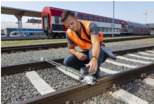
Rail geometry measurement with the multifunctional CALIPRI measuring gauge
