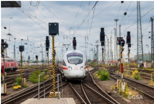
Track & signalling site
