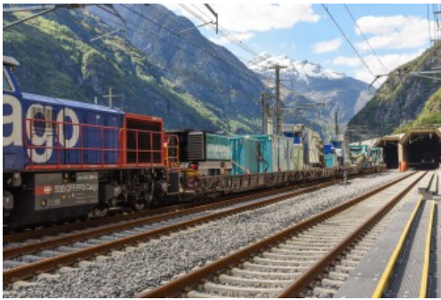
Cleaning train with various components
