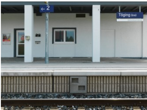
Highly absorbent platform edge in Töging am Inn
