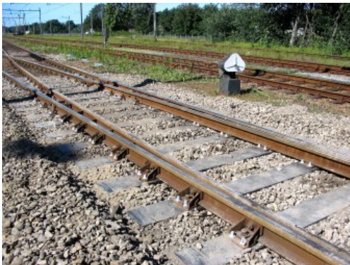
KLP® Hybrid Polymer Sleepers for Corus-Tata Steel IJmuiden
