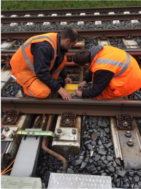
LAT technicians install sensor technology in track bed
