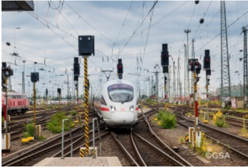
Track & signalling site
