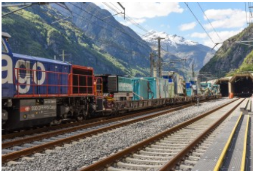
Cleaning train with various components
