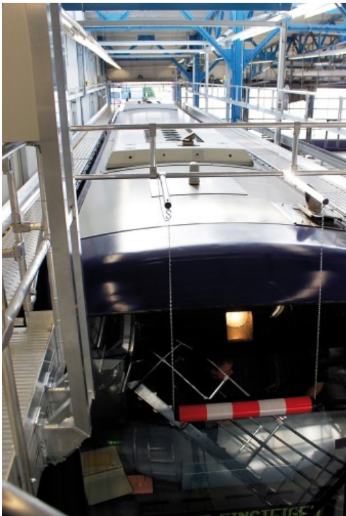
Front side guardrail, platform with ramming protection still retracted
