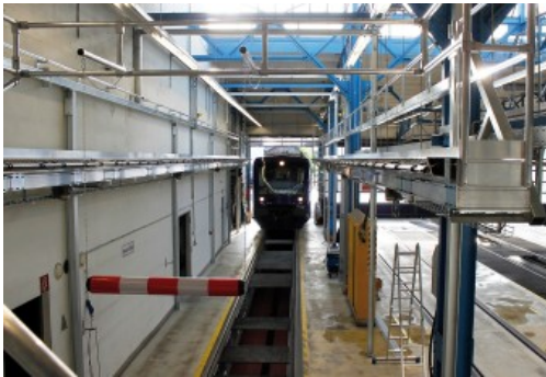
Entry of the train; platform retracted with impact protection, additional visual distance stop
